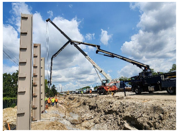
Noise wall construction continues along the Central Tri-State Tollway (I-294). Westchester
