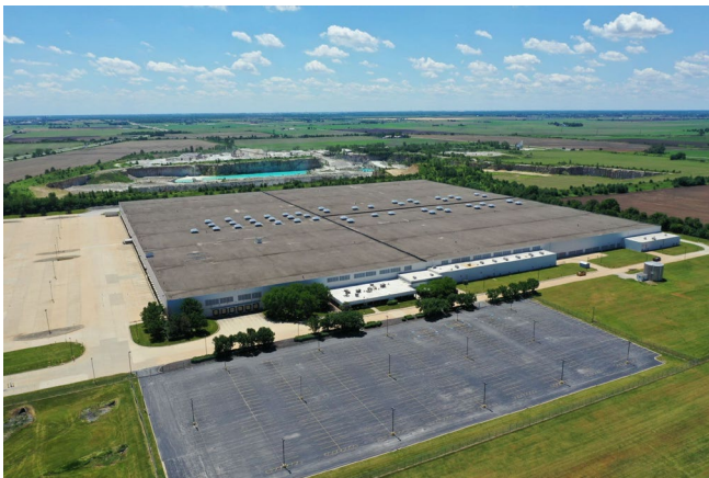
Exterior view of planned Gotion plant. from north-east. Manteno.
