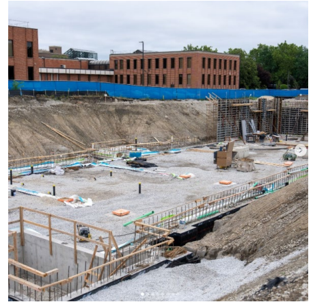
Foundation work for Education Building at Northeastern Illinois University. Chicago.
