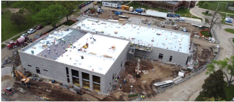
New plant at Elgin Mental Health, exterior view. Elgin.
