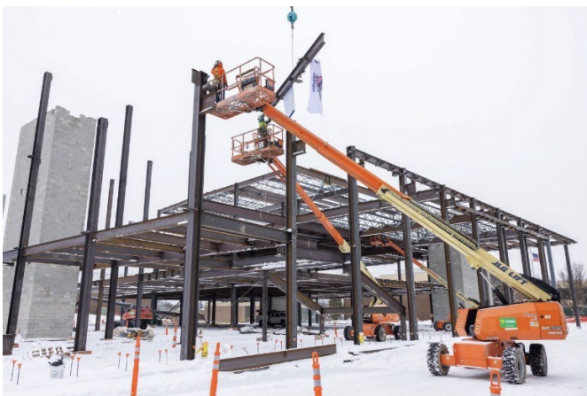
Construction of the Canning Student Center and University Center. Palatine.
