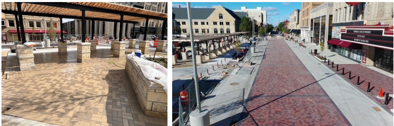
Infrastructure improvements outside of Rialto Square Theater as of October 2025. Joliet.
