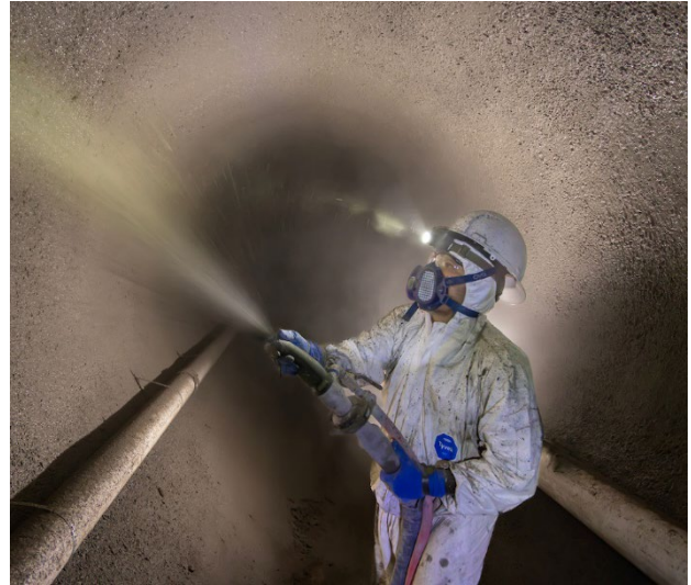
Combined sewer rehabilitation. Lombard.
