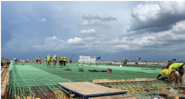
Bridge deck work for the new I-490/I-90 Interchange near Des Plaines
