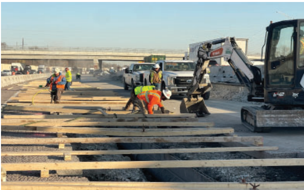
Roadway reconstruction along the Central Tri-State Tollway (I-294) near Hinsdale.
